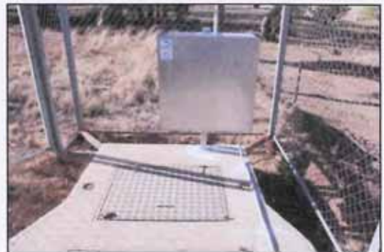
Aabove: Bacteria dosing cabinet at pumping station
