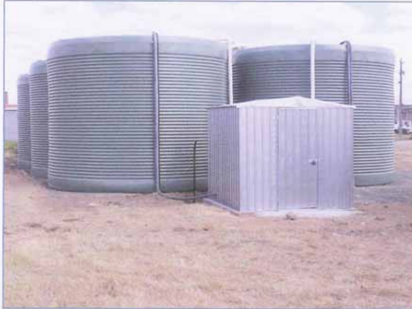
Sample Photo of 3 tank system.
