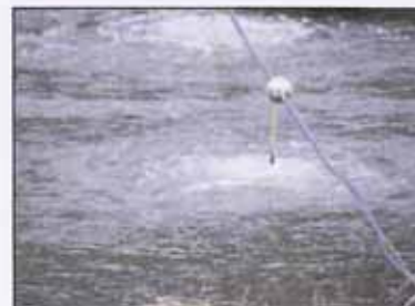
Aeration line suspended by stainless cable. Air stones set at various depths to follow dam bottom.
