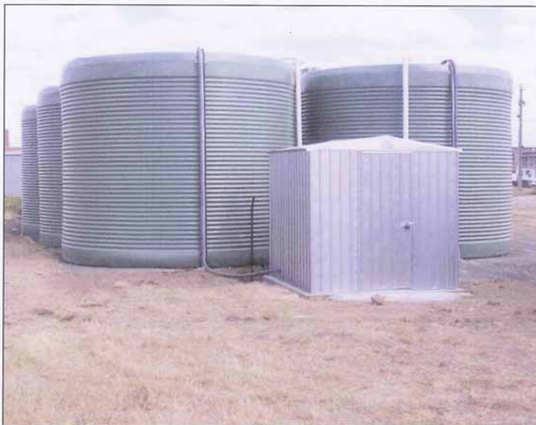
Three tank bio-reactor system – Ballarat Saleyard.
