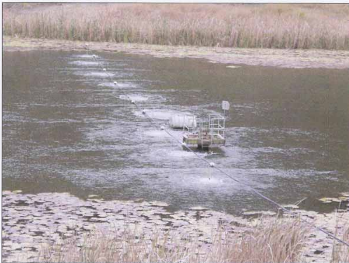
Aeration line suspended by stainless cable. Air stones set at various depths to follow dam bottom.
