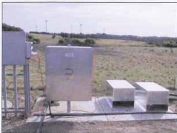
Bacteria Dosing Cabinet and aeration pumps
